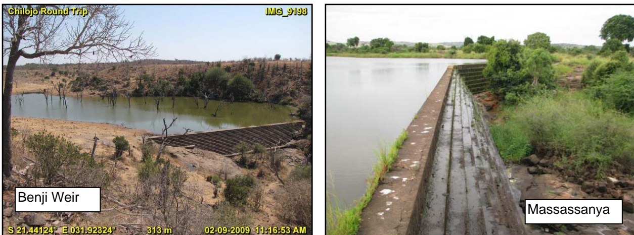
Figure 14: The two Gonarezhou weirs
